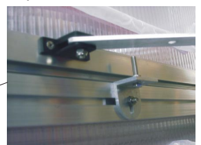
Window fixing with screw 4,2x16 to screw down
